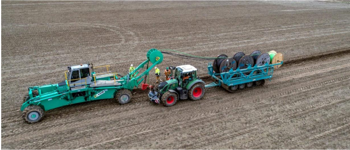
Plate 2: An example photo of cable ploughing
