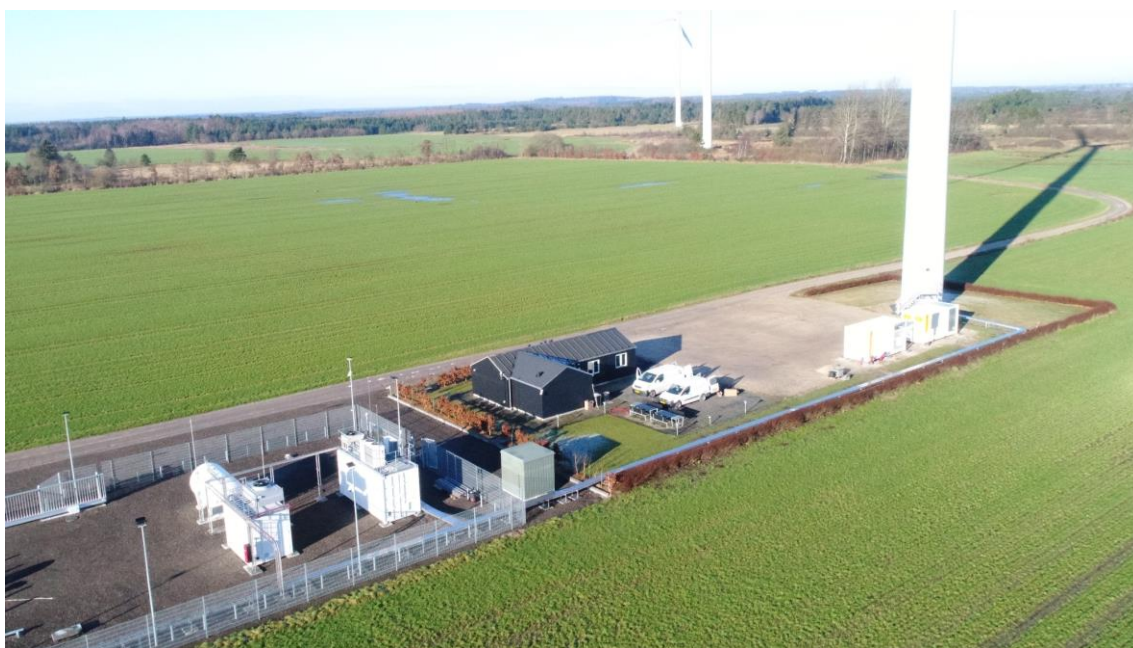
Plate 1: An example of a small-scale Green Hydrogen Facility in Denmark
