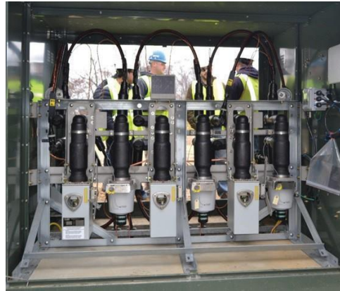
Figure 12: G&W Viper Recloser With G&W Trident Bypass and the Three-Line Diagram
