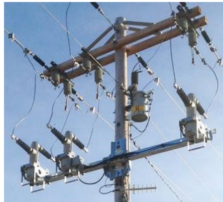
Figure 9: G&W Viper Recloser With Z-Shaped Modules and Extended Phase Spacing
